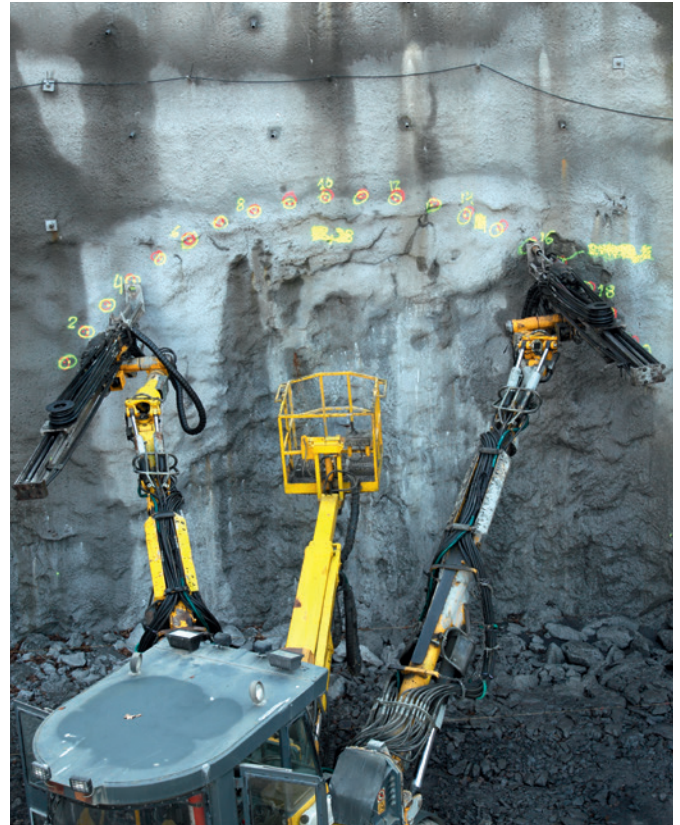
Pipe roofing application with a boomer.
