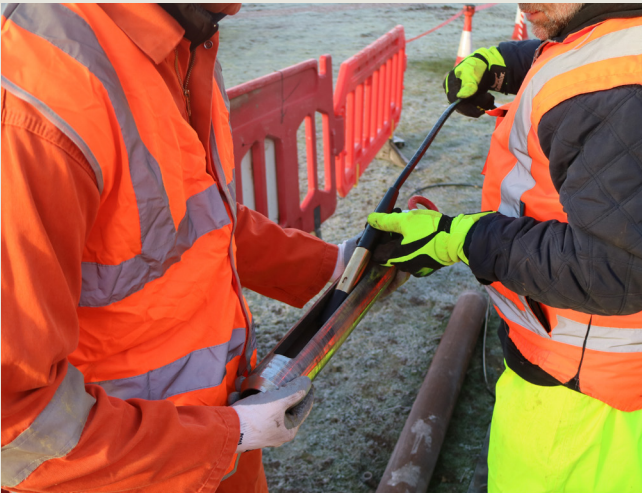
Building up the tool from the top
