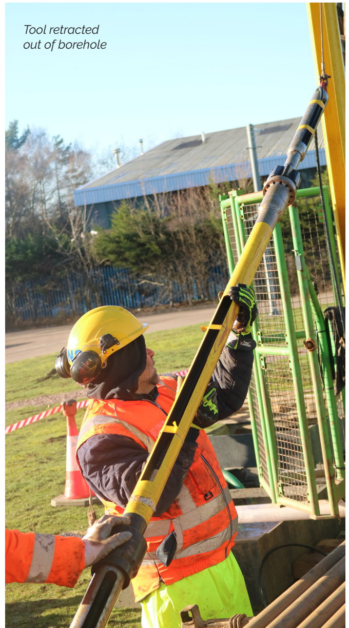
Pushing the drill string into the test pocket
