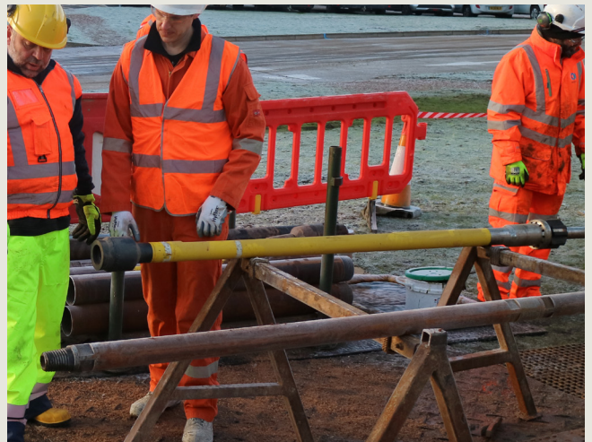
Connecting the tool to the HPD
